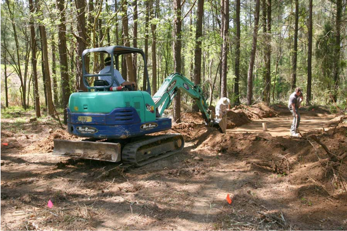
Figure 3.15. Removing flood sands and modern plowed soil with a trackhoe during phase I stripping at the Ashe Ferry site.
