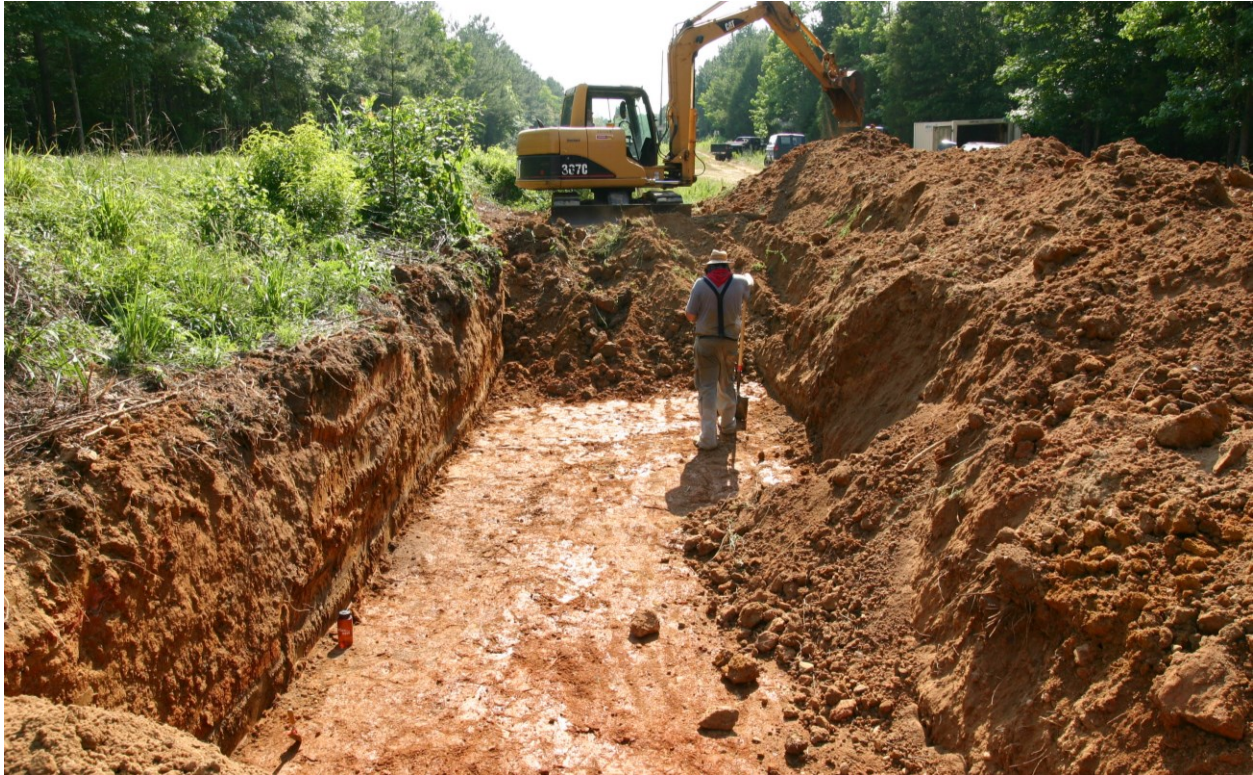
Figure 3.14. Exposing the top of subsoil surface near the SC Highway 5 embankment. View to west.
