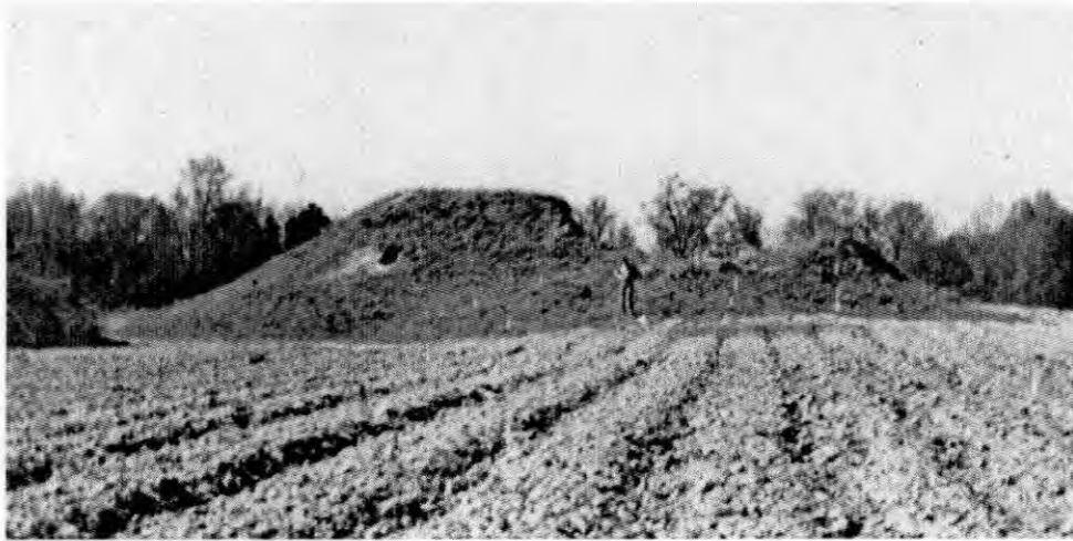
Figure 1.9. 1937 photograph showing damage to the eastern part of the Town Creek mound (RLA negative X2349).
