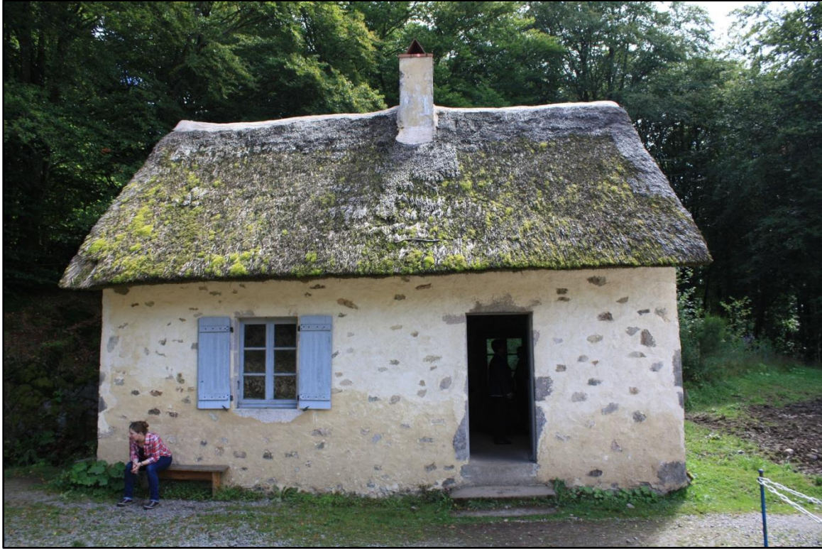
Figure 6.1. On-site reconstruction of the “ Hôtel des Gaules ,” the house built by Jacques Gabriel Bulliot on the summit of Mont Beuvray in 1870.
