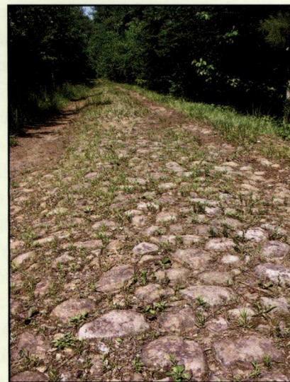
The cobblestone roadbed known as the Old Oxford Road, or New Hope Road, passes through the Duke Forest. Duke Forest Photo Collection.
