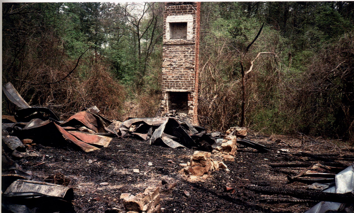
All that remains of the Nettie Couch house. Lightning likely struck the abandoned home in the late 1980s. Duke Forest Photo Collection.
